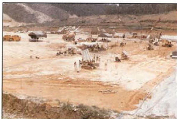
Fig. 14. Foundation grouting at Batu Dam, K.L.
