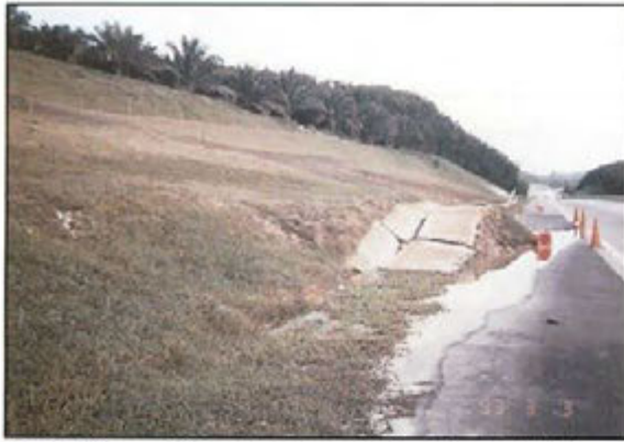
Fig. 7. "Flattened" cut slope in graphitic schist, N-S Highway near Rawang.
