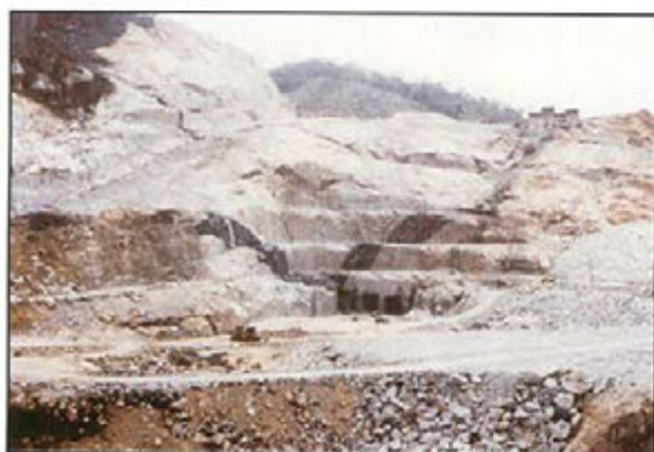
Fig. 15. Kenyir Dam, a rockfill dam, Kuala Berang, Terengganu. Dolerite dykes (black) in granite.
