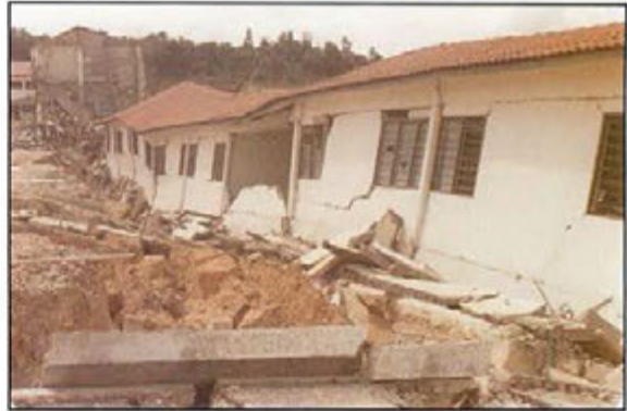
Fig. 12. Rapid draw-down of mining pond triggering slope failure and destroying houses, Kuala Lumpur.
