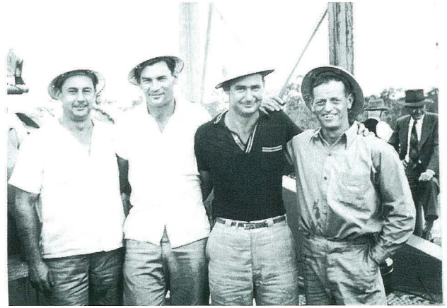
OD&E's first drilling crew – Jock Weir, Pete Brewster, Jay Gray Sonny Westphal (Roger Watson in background at right) – all from the USA – at the spudding ceremony of the company's first well, Cherwell Creek#1. The rig used was at National 80B, designated Rig#1.
