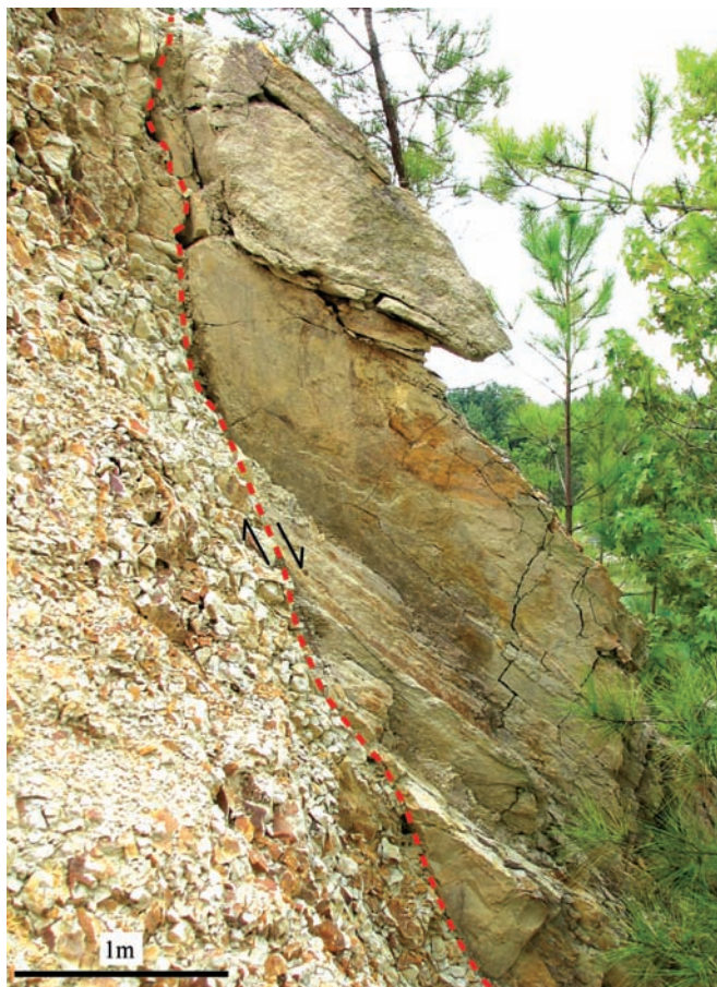
Figure 5: Cross section of a NNW-trending normal fault showing juxtaposed sandstone against underlying clay deposit.
