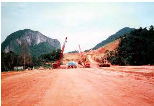
Figure1: North-South Highway under construction, looking north. G. Tempurung (limestone) on the left, schist in cut-slope on the right, and granite further right (Main Range). Colluvium occurs along the Highway mainly as valley fills.
