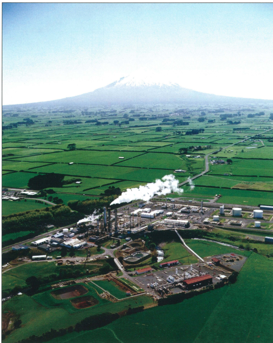
The Kapuni processing plant. The Kapuni field has been in constant production since 1969.
