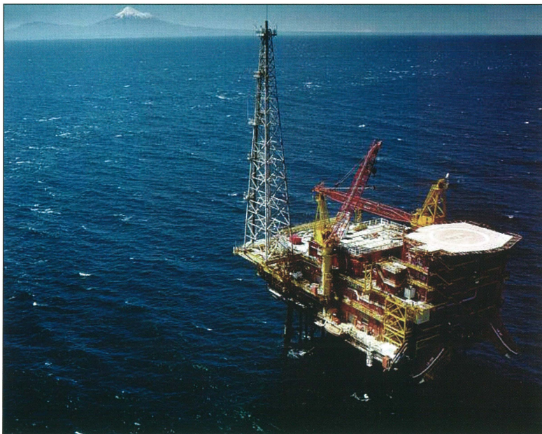
One of two platforms in the Maui field, Maui A has been in production since 1979.
