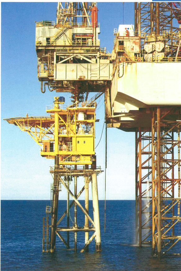
Jack-up drill rig over John Brookes wellhead, Carnarvon Basin, Western Australia.
