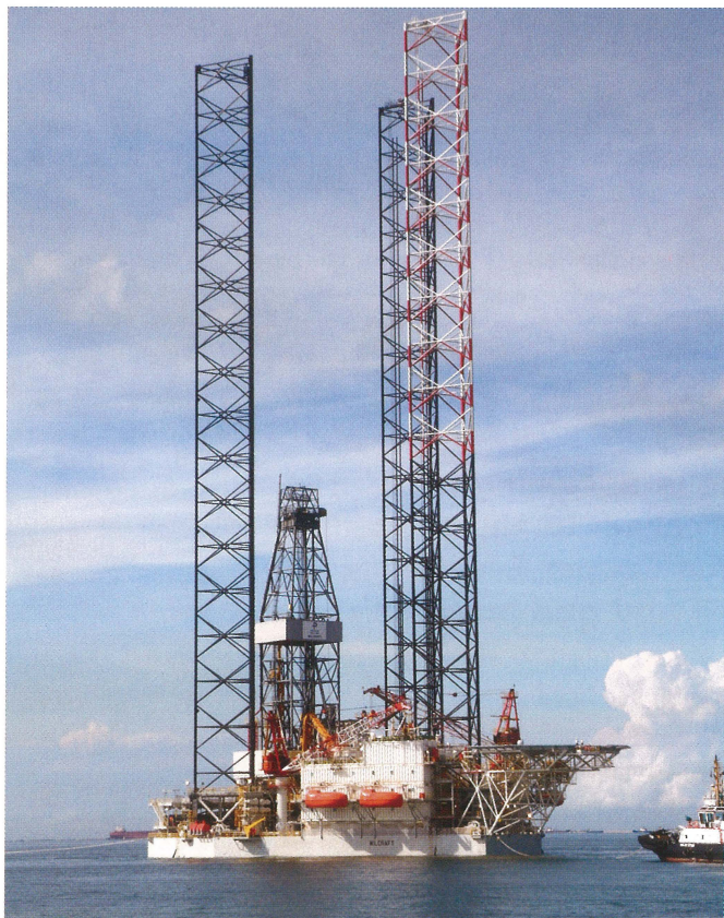
The brand new ultra Premium Wilcraft jack up rig was commissioned by Awilco Offshore in December 2006 and is capable of drilling in water depths up to 122 m and to drill high pressure and high temperature wells down to 9,144 m drilling depth. The rig is on a 13-24 month contract with the AGR Group for work offshore Australia.
