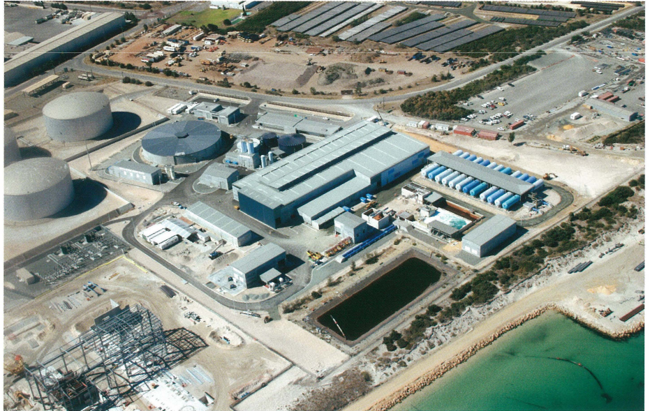
The Kwinana sea water desalination plant has demonstrated that large quantities of water from an unlimited ocean supply can be provided using a clean and green process.
